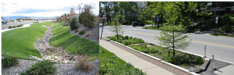
Bioretention Basins / Rain Gardens
